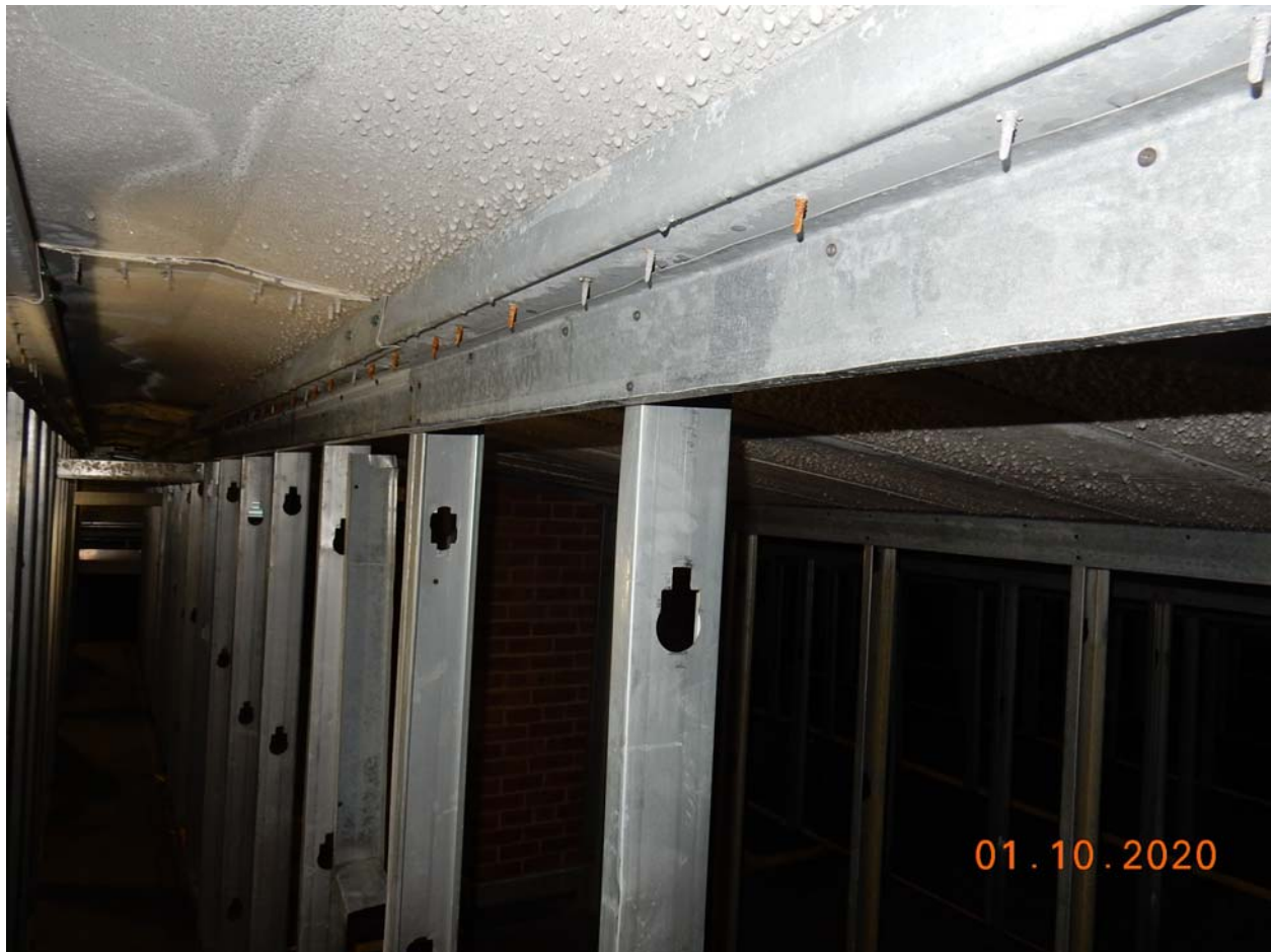
Looking south in attic space near south end of classroom wing, directly under ridge cap. Rows of studs at right are in southwest quadrant of attic and are reinforced with strongback (another track section). Note condensation on underside of ridge cap and standing seam roofing to right.
